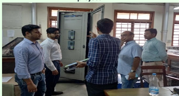
Numerical Relay in the Power System Protection Lab
